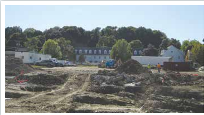
Construction on the new medical center at the old Danbury Police Department site on Main St.
