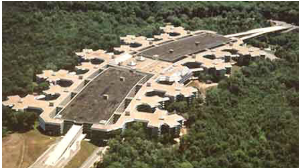
THE MATRIX CORPORATE CENTER DANBURY WEST SIDE 1,300,000 SQUARE FEET
