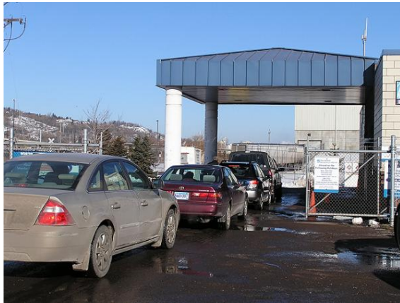
HHW PERMANENT FACILITY
